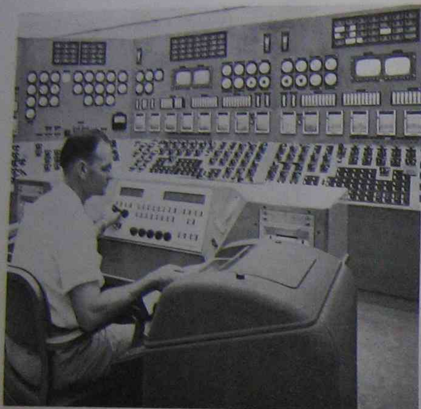
GEORGIA POWER COMPANY'S McDonough plant uses digital computer to monitor two 250-mw units. Operator inserts fuel analysis data to obtain continuous record of heat rate.
