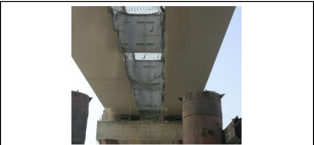
Figure 3.6-2 Safety Net between Scaffold Plates
