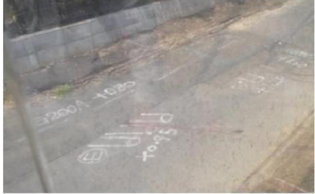
Figure 4.1-3 Buried Position Marker (Road Surface)
