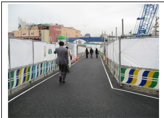
Figure 3.2-1 Guard Fence and Sheet 1
