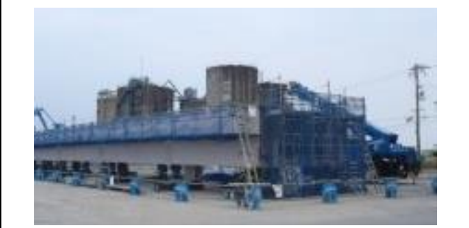
Figure 10.3-1 Assembly Work at Ground
