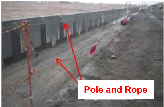
Figure 3.5-8 Fall Prevention at top of Slope
