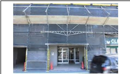
Figure 3.6-1 Flying and Falling Objects Prevention at Entrance
