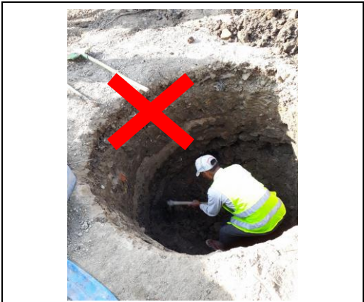
Figure 8.1-1 Fall Prevention for Pile Hole
