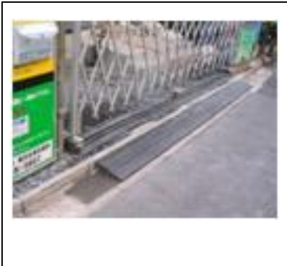
Figure 3.2-6 Elimination of a Level of Difference
