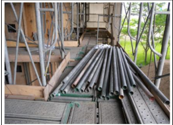
Figure 3.6-5 Not to put materials on scaffolding
