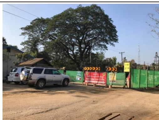
Figure 3.2-2 Guard Fence and Sheet 2
