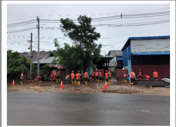
Figure 3.1-1 Proper Equipment (All site)
