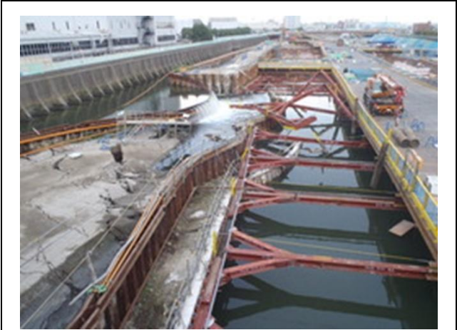
Figure 6.3-1 Temporary Cofferdam
