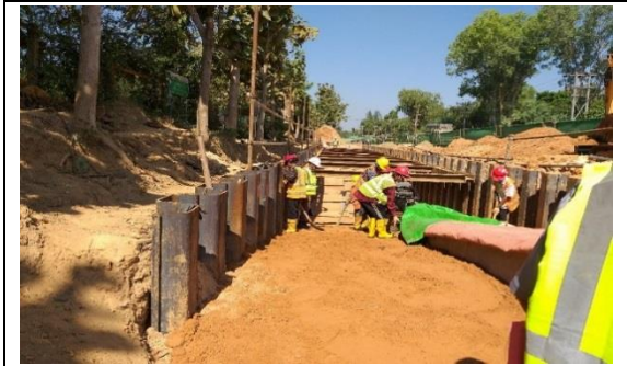
Figure 6.2-1 Earth Retaining Construction
