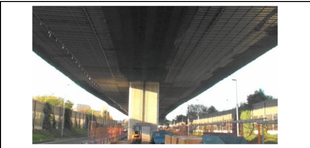
Figure 3.6-3 Flying and Falling Objects Prevention at the site close to existing road
