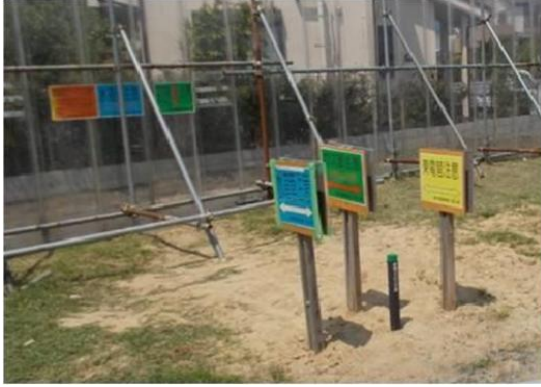
Figure 4.1-2 Buried Position Marker
