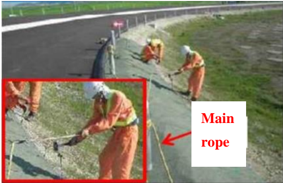
Figure 3.5-6 Main Rope and Safety Belts
