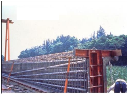
Setting of Re-bars and PC tendon
