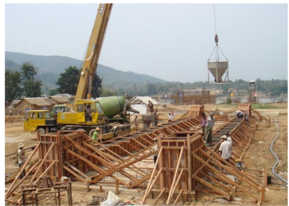
Construction of Strut Beam
