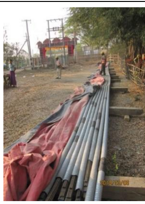
2.1-2 Storage of ducts and PC steel
