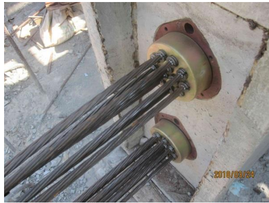
2.2-2 Anchor head before prestressing
