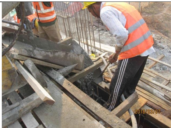
2.1-15 Concrete casting (2)
