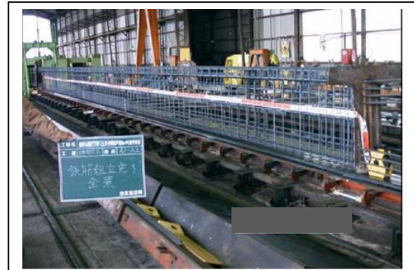
Setting of reinforcing bars
