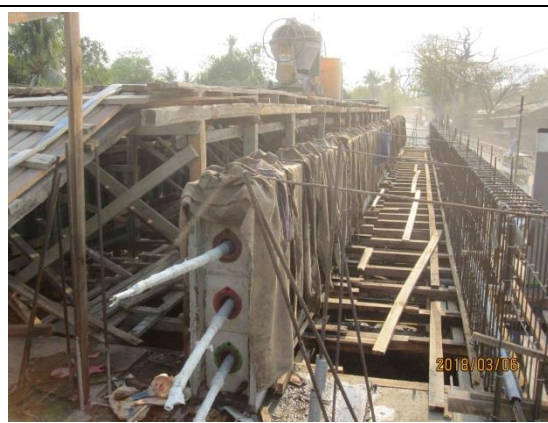
2.1-16 Curing of concrete
