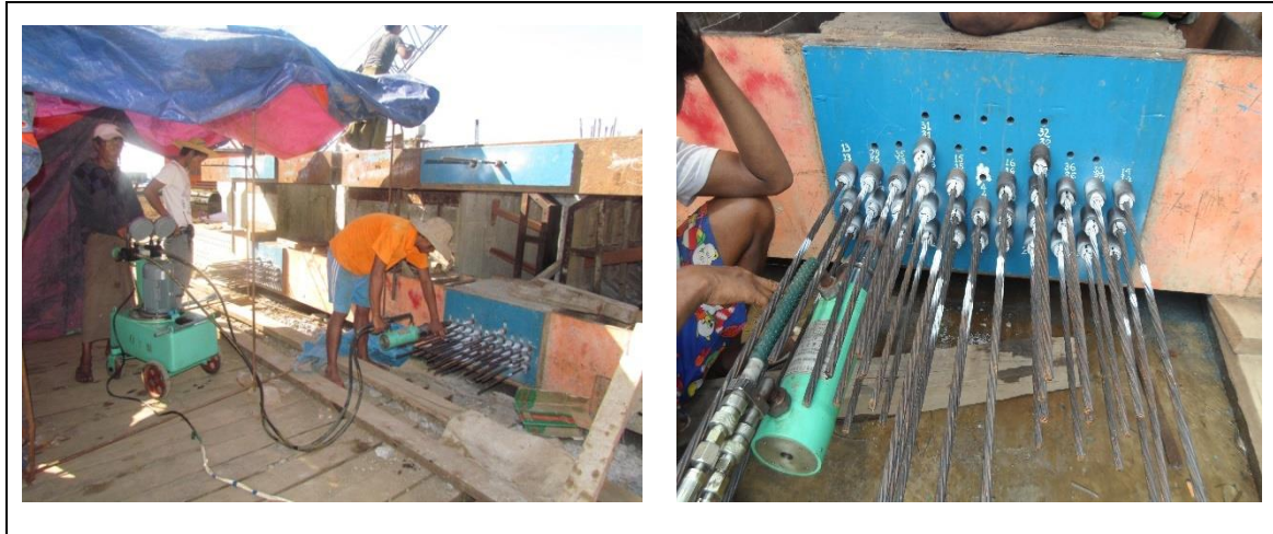
Figure 8.3-1 Tensioning of Pre-tensioning Material (Site Product)
