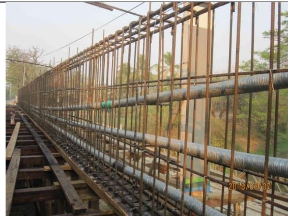
2.1-3 Setting of rebar and ducts
