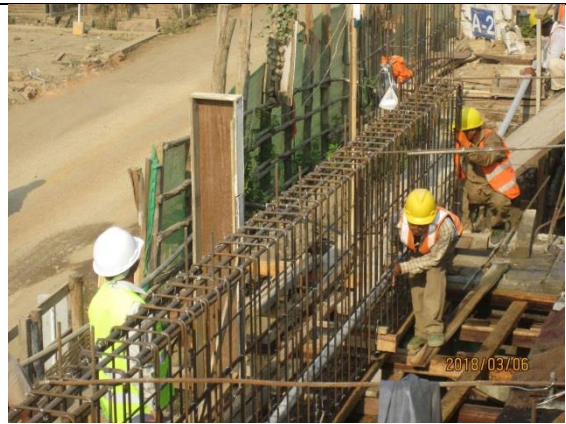
2.1-4 Setting of duct
