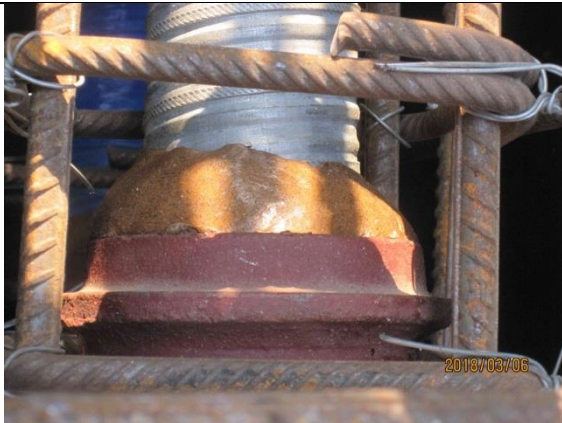
2.1-11 Sealing between duct and anchorage
