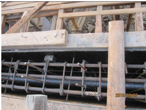
2.1-7 Division number of ducts shall be odd number
