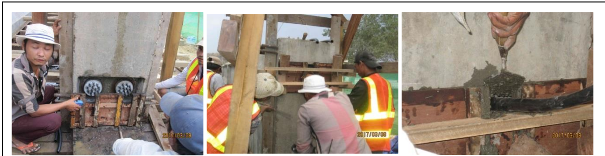
Figure 9.9-1 Protection of End Anchorage in Myanmar
