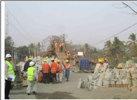
2.1-1 View of the work site
