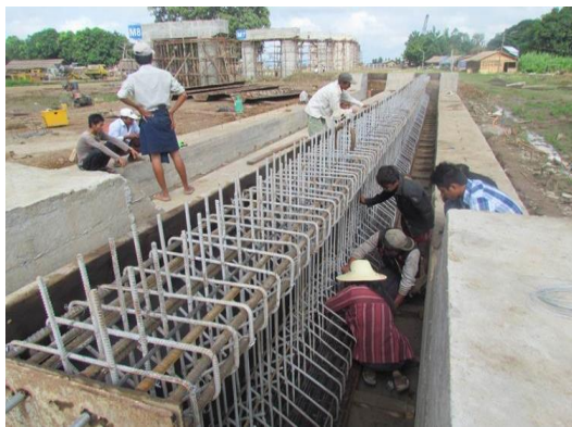
Steel Reinforcement Fixing
