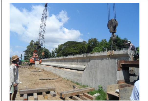
Figure 8.1-2 Prestressing Equipment (Strut Beam) for Post-Tension Girder (At the Site)
