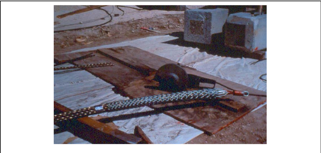
Figure 3.2-1 Steel Wire Sock for Installing Multi-strand Tendon
