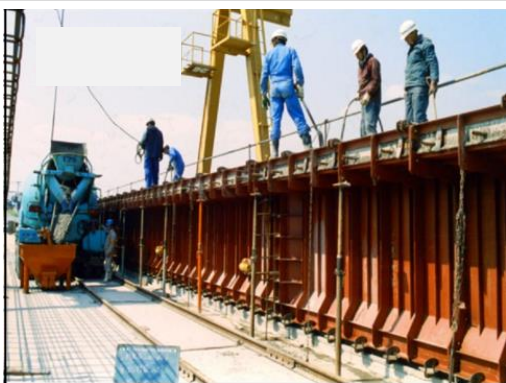
Casting of concrete
