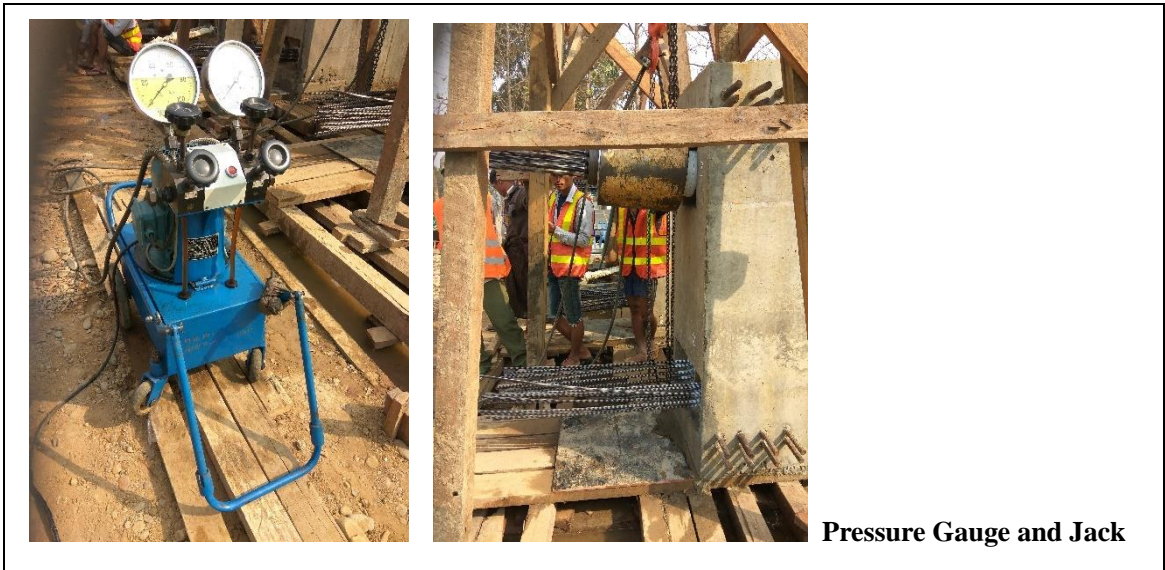
Figure 8.1-3 Prestressing Equipment for Post-Tension Girder
