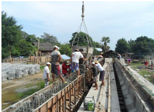
Concreting of Girder
