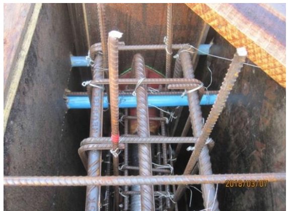
2.1-10 Duct and anchorage
