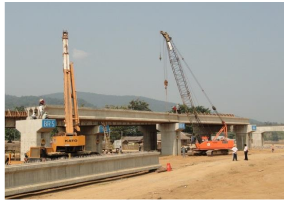
Placing of PC Girder
