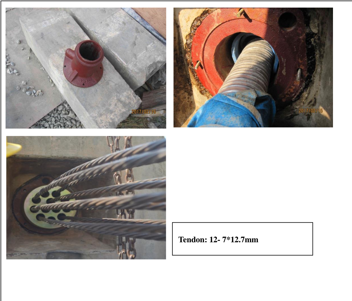
Figure 2.2-2 Typical Anchorage in Myanmar
