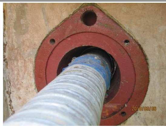
2.1-12 End duct at anchorage (after casting concrete)
