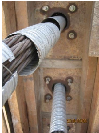
2.1-13 End duct at anchorage (before casting concrete)
