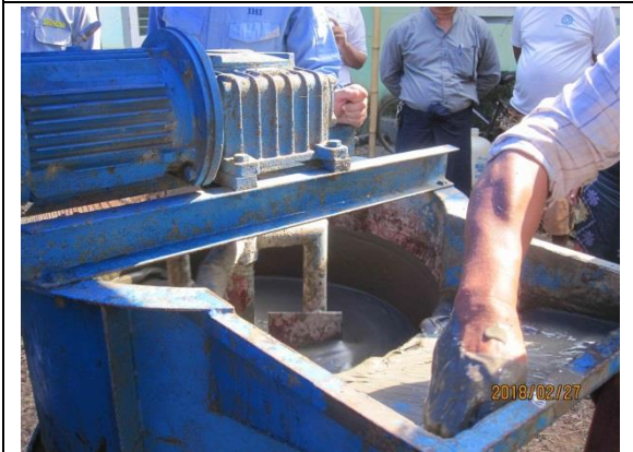
1.1-3 Slow mixing hopper to pump
