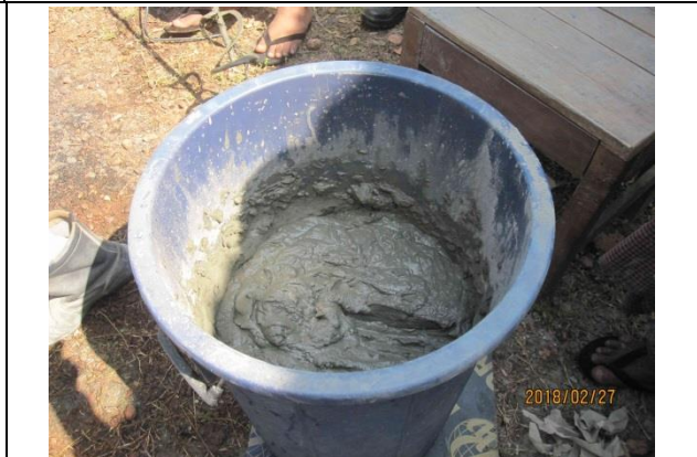
1.1-4 Bad mixing of APT (not available for testing)
