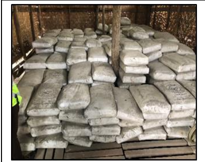
Figure 6.1-2 Recommendable Plan for Storage of Cement Bags
