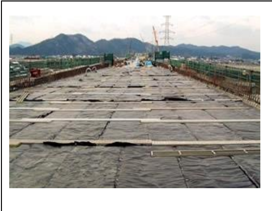
Figure 10.1-1 Wet Curing Sheet
